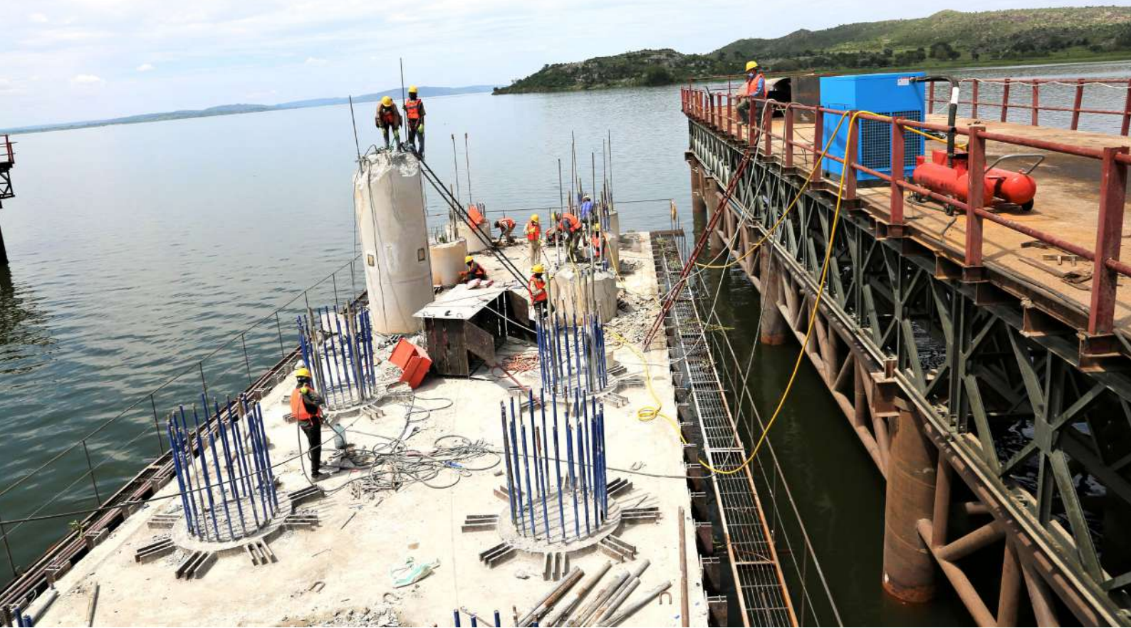
The Work on the construction of the foundation pillars of the JPM (Kigongo - Busisi) Bridge continues in Mwanza Region.
